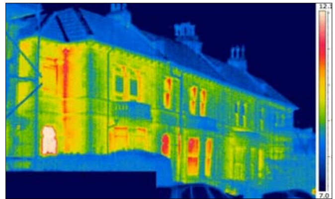
Thermographic imaging of existing terraces to identify heat loss 'cold spots'
