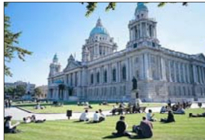
Belfast City Hall - £3m refurbishment including full services renewal to reduce CO 2 emissions
